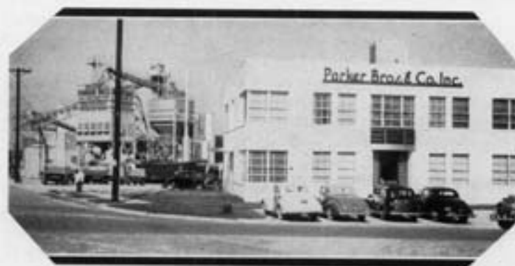
Home of Parker Bros. Shell Building Material and Ready-Mixed Concrete.
