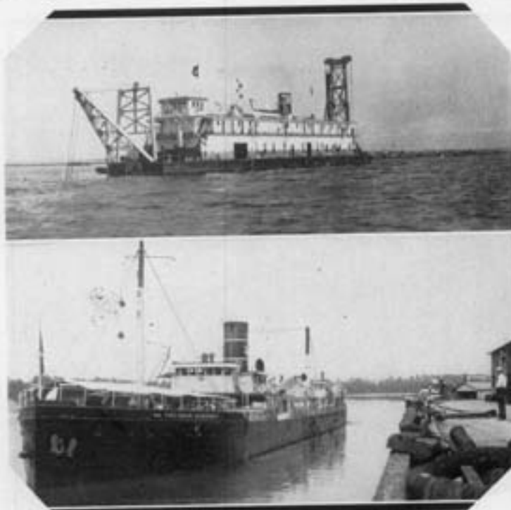
TOP: U. S. Dredge Raymond maintaining bay section of the Houston Ship Channel. BOTTOM: U. S. Seagoing Hopper Dredge Galveston on emergency work in Channel.
