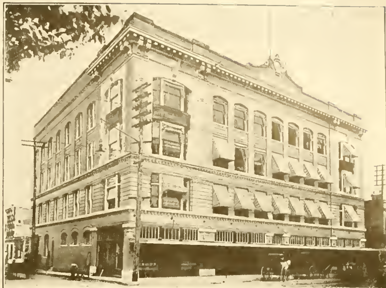
Prudential Building. —Atlee B. Ayres, Architect.
