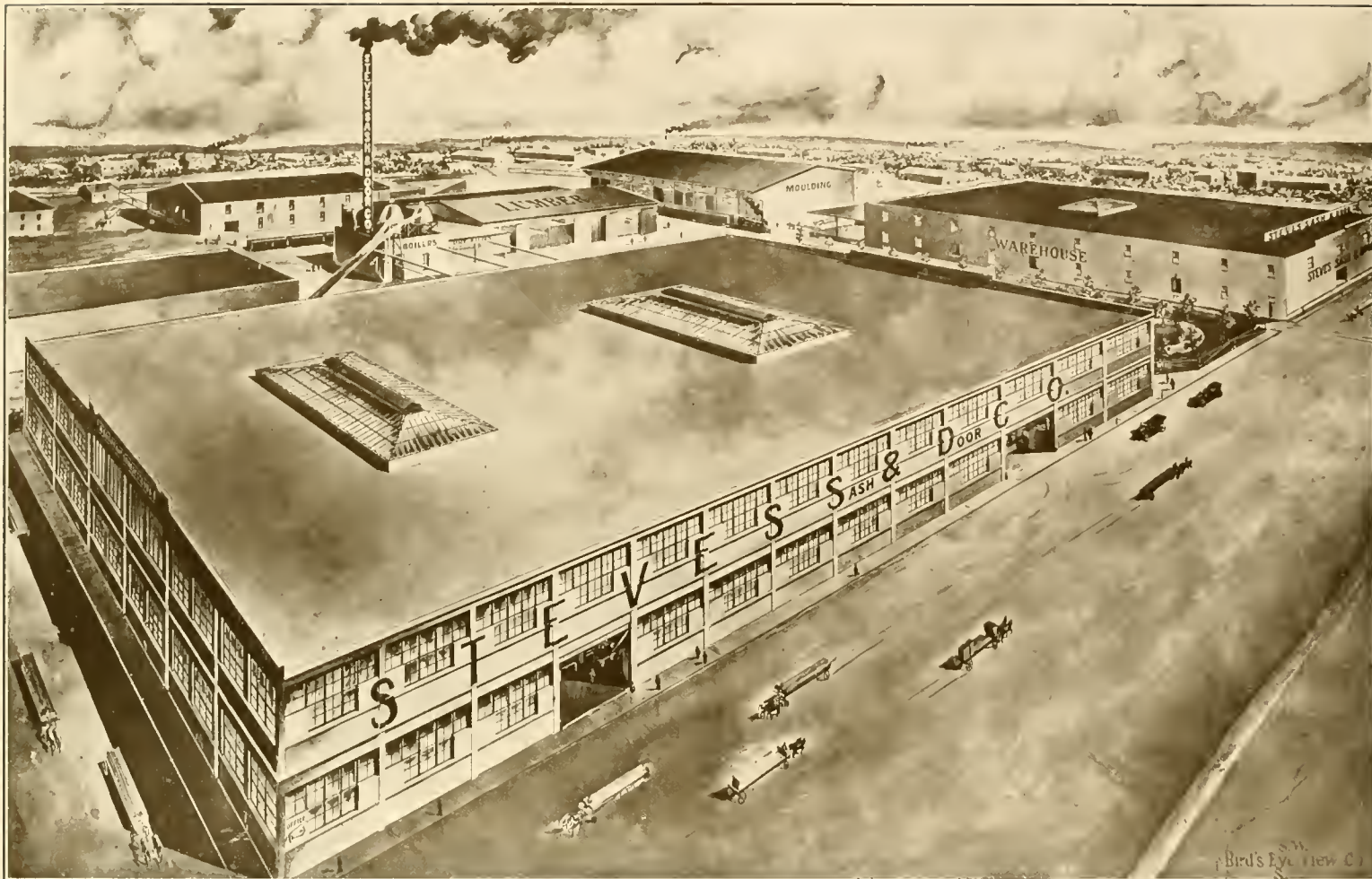
Steves Sash and Door Company.
