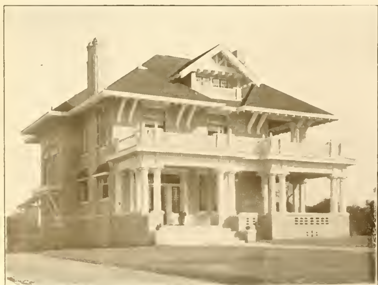
Residence R. Surkamp.
