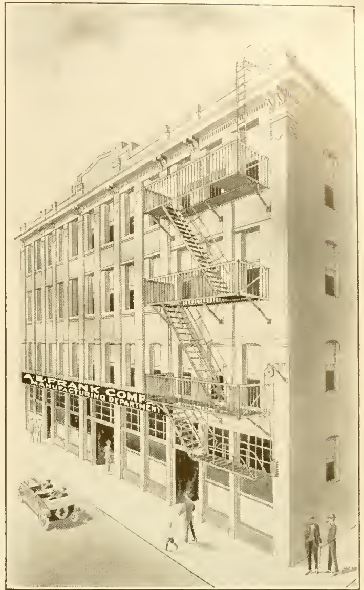
A. B. Frank Company. —Atlee B. Ayres, Architect.
