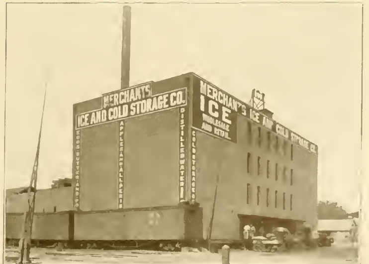
Merchants' Ice and Cold Storage Company.
