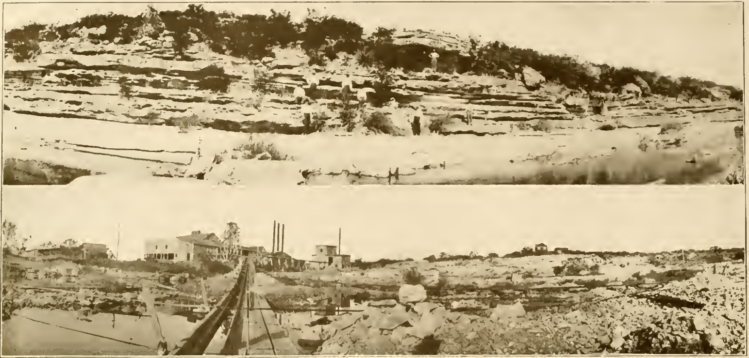
Numerous Streets in San Antonio Are Paved With This Material.
