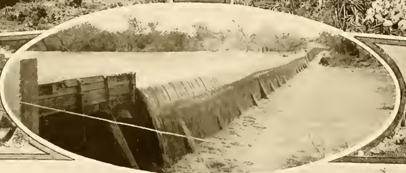
DAM IN FRIO RIVER AT FOWLETON
