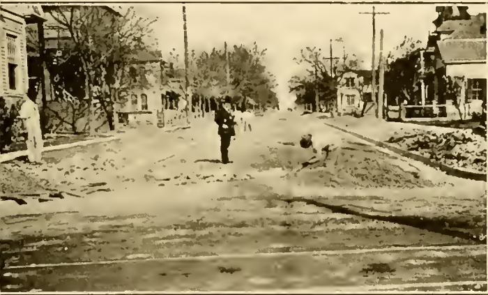
Construction of a Trap Rock Road.
