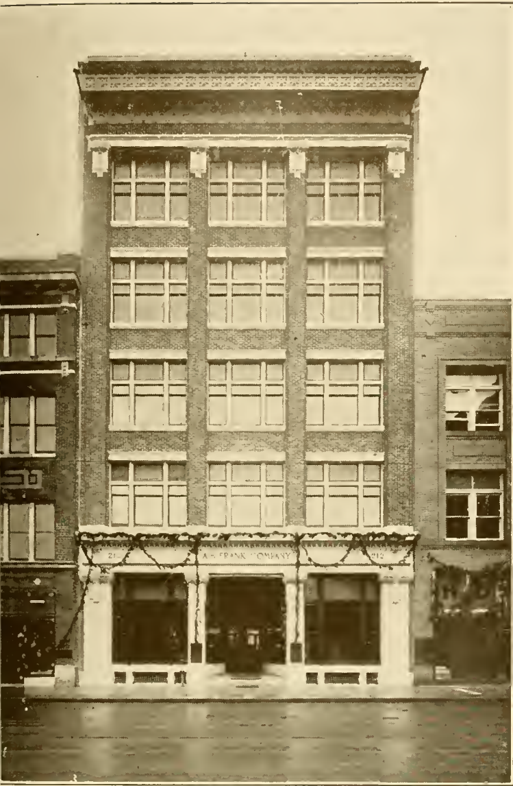
A. B. Frank Company. —Atlee B. Ayres, Architect.
